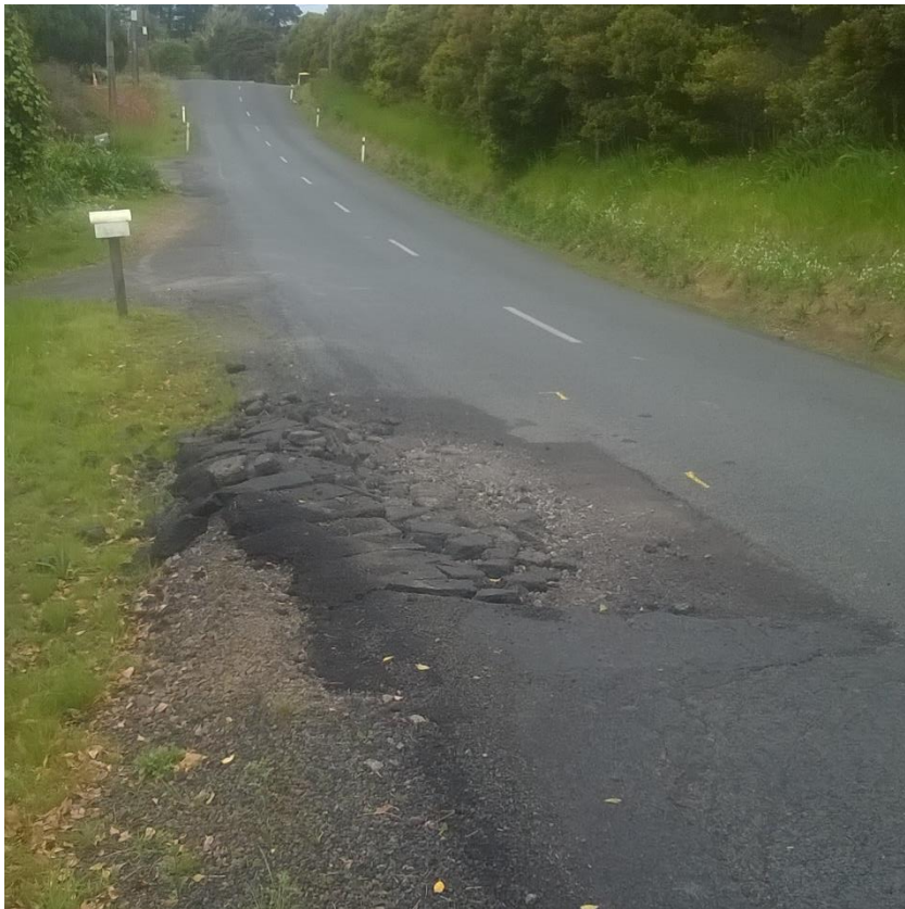
Figure 2: Rural Road Failure on a Cleanfill Project
