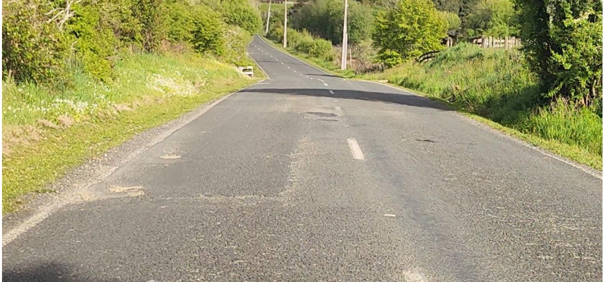
CH16060 to CH 16130, east bound lane. Scabbing.
