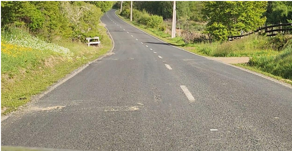
CH 15910 to 16020, West bound lane. Previous repair rutting on edges and inside wheel path.
