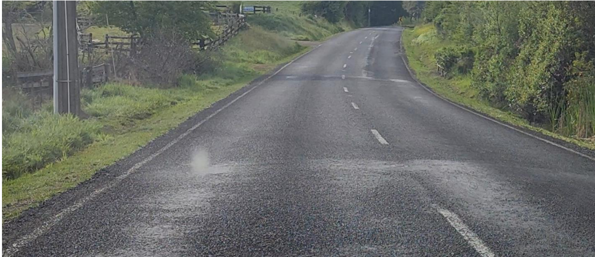
CH 15910 to 16020, West bound lane. Previous repair rutting on edges and inside wheel path.
