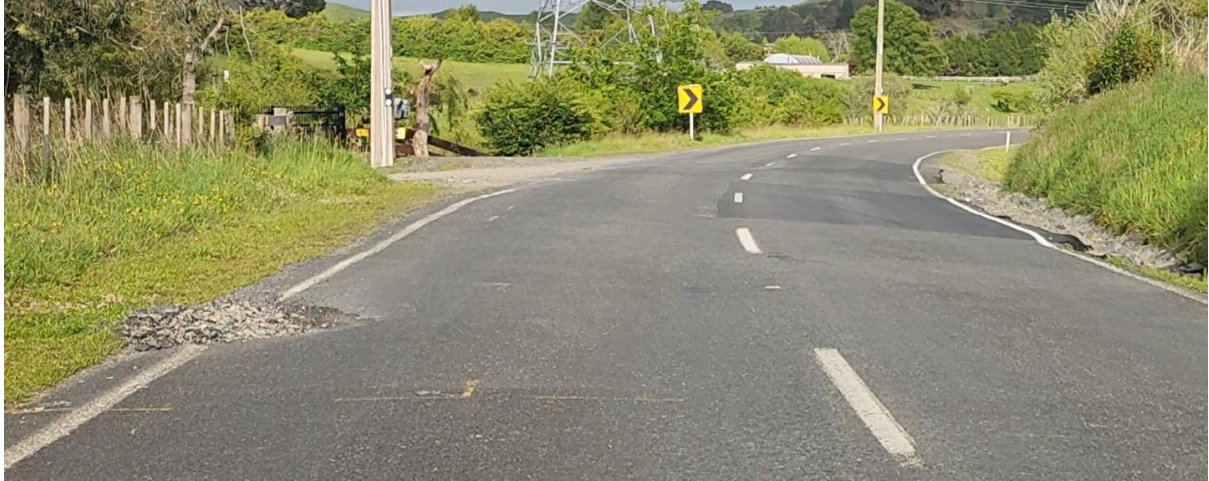
CH16535, west bound lane, Pothole and shoving, east bound lane rutting in wheel path.
