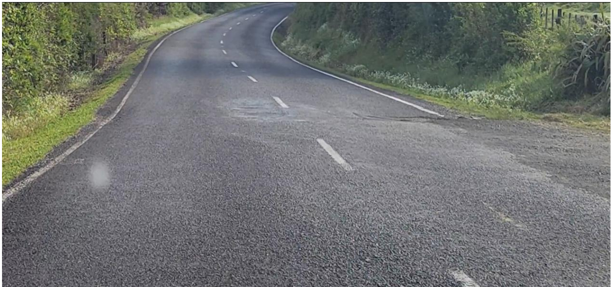
CH 16610 and CH 16700– Rutting in wheel path, east bound lane.
