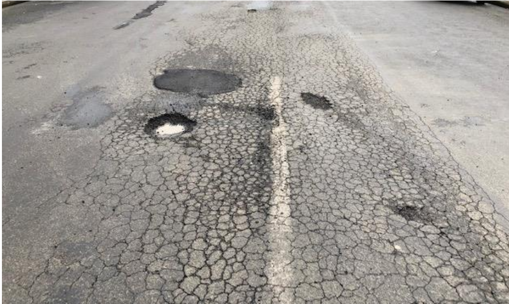
Figure 1: Urban Road Failure on a Housing Development Project
